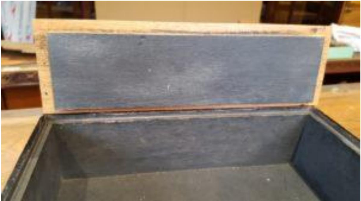
4 Lid partly constructed showing the shrinkage in keeping with the original section.
