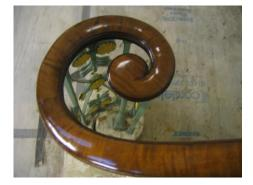
With the entire handrail in position, terminals in place, end sections carved and any remaining inserts put back into place, the remaining original patination was preserved, and sections of inserts, and any newly created areas, patinated to blend in.
