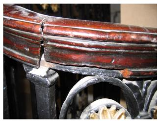
Necessary repairs to the handrail were then undertaken including having to re-build all of the corner sections, which were badly damaged and to replace two sections of handrail (previously badly repaired).
